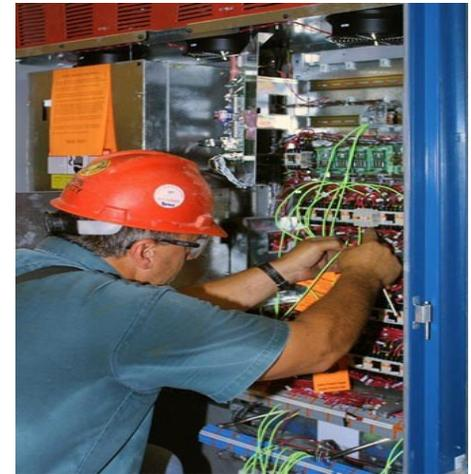
Relay logic or PLC control wiring and panels must be restored including partially rewiring, replacement of micro-circuitry and sensitive relays, contacts and din rails prior to being tested and put back into service. It is important that professionals work on these technical aspects of the claim from beginning to end to ensure that the systems are inventoried, restored, tested and put back into service with track ability.
