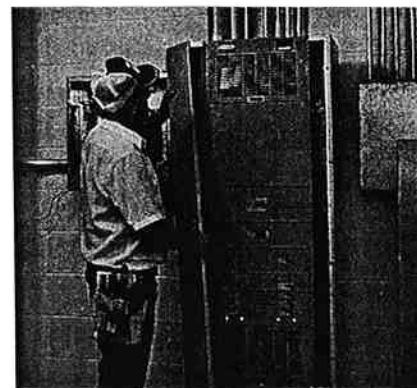
The three-piece trim for larger power distribution panelboards provides for easy handling and installation
